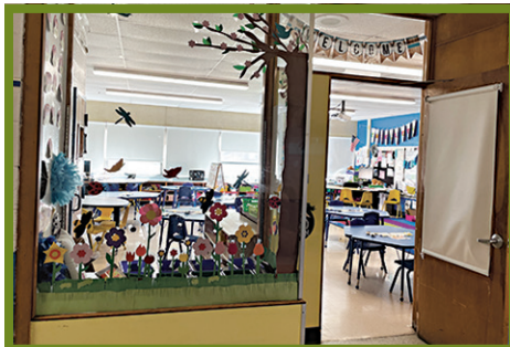
The original "storefront" window designs at Monticello elementary schools. The proposed capital improvement project would replace these entrances with more secure, fire-resistant and reinforced classroom doors.
